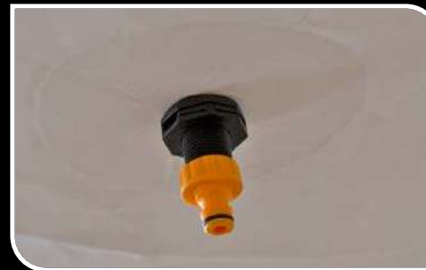
Central Drainage Point
